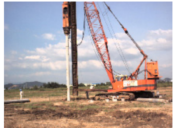
Figure 9. Driving pile into ground
